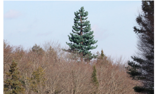
Bell certifies that all its antenna base-station installations or towers meet or exceed federal Safety Code 6 requirements. In this picture a tower is disguised as a tree and is positioned to blend with the environment.
