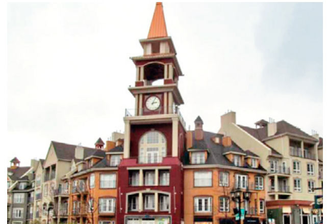
In this picture, a cellular antenna is embedded in a clock tower.
