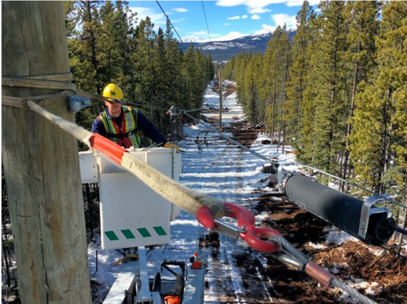
In this picture, technician Burt Stephens and crew are working on a series of pole transfers near Carcross Yukon.
