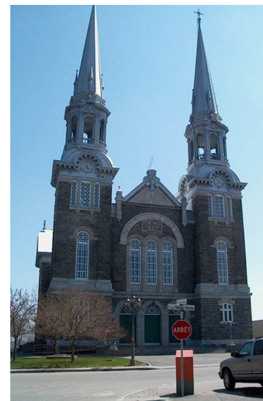
A series of antennas are camouflaged inside the bell tower, whose arrow has been modified to include 2 antennas pointing in 2 directions in a church on Notre-Dame street, Ancienne Lorette, Québec.
