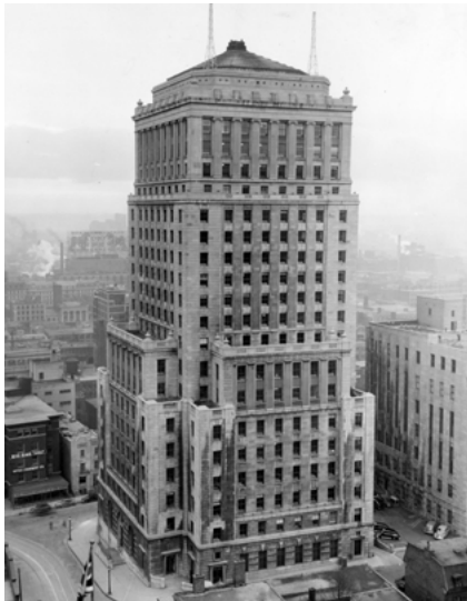
For more than 80 years, starting in 1929, Bell's head office was at 1050 Beaver Hall Hill, in Montréal.
